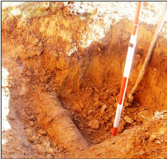
Plate 13. Area dug for silt trap north side of building. Clay pipe became visible running alongside the buildings north wall. View west.
