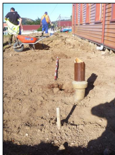
Plate 17. Upright lead pipe and clay pipe of lean-to. View south.
