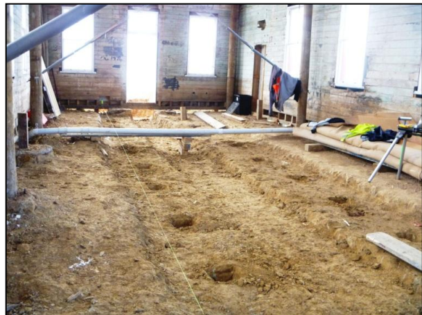
Plate 8. New post holes dug for new piles.
