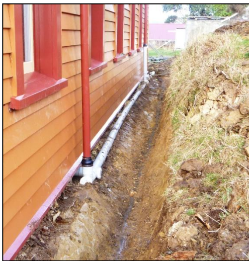
Plate 11. Drain coil in base of re-dug trench rear wall. View south.
