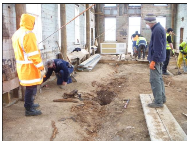
Plate 5. Post hole 5.4m north (west bearer) visible once bearer lifted.
