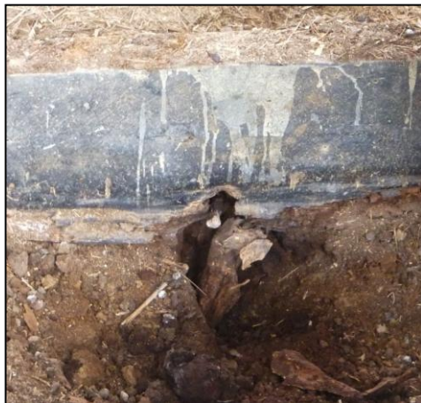
Plate 7. Remnant pile and cut nail beneath bearer 7.4m north Section E (item 20).
